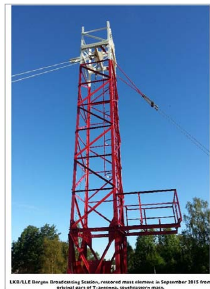
LKR/LLE Bergen Broadcasting Station, restored mast element in September 2015 from original parts of T-antenna, southeastern mast.
